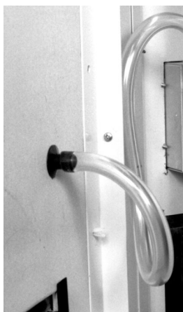
Figure 4: Back view of fascia
