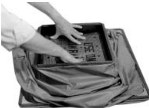
Figure 6: Installation of LoFlow screen
